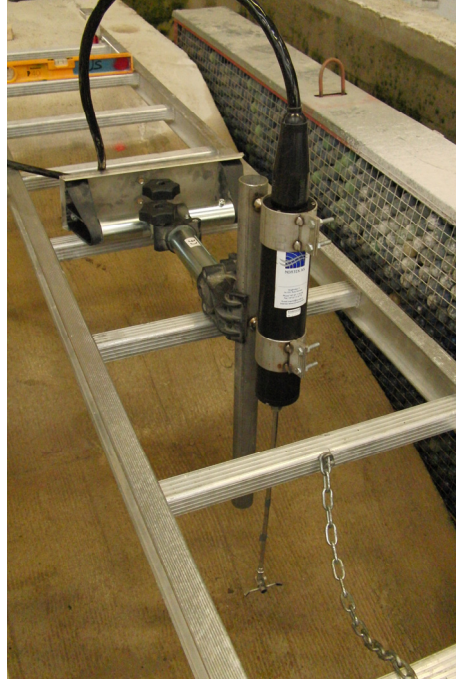
Figure 2: Acoustic measuring probe mounted in place
