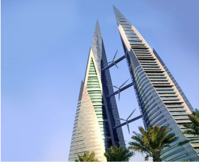
Figure 1: Three integrated horizontal axis wind turbines between the Bahrain World Trade Center skyscrapers (WWW)
