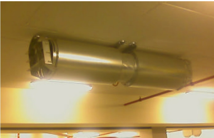
Figure 2 - Jet fan in an underground car park and numerical jet fan model.
